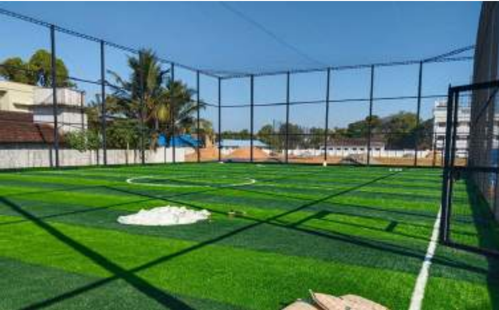
Futsal works ongoing
